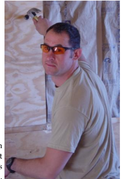
SSG Jason Arsenault hangs sheets of plywood.
